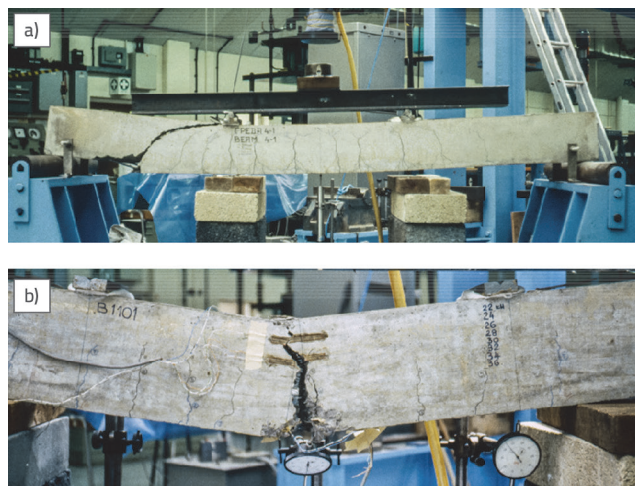
Figure 11. Failure mode of: a) RB-PC beams; b) RB-SF beams
